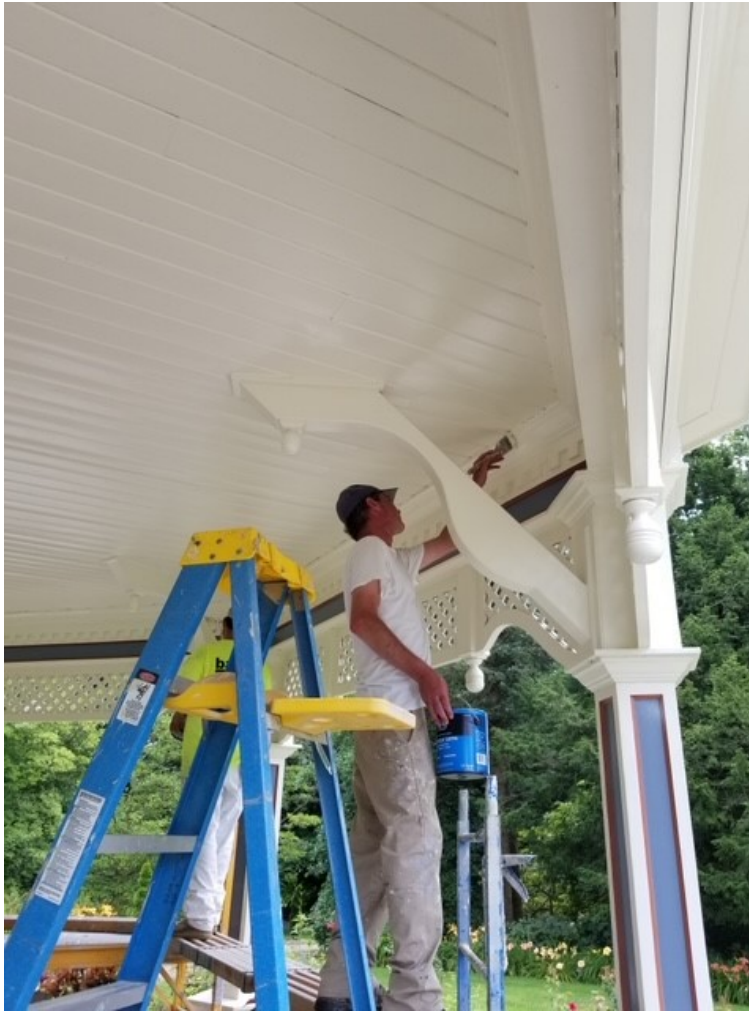
Gazebo Pavilion Painting project - 2019
