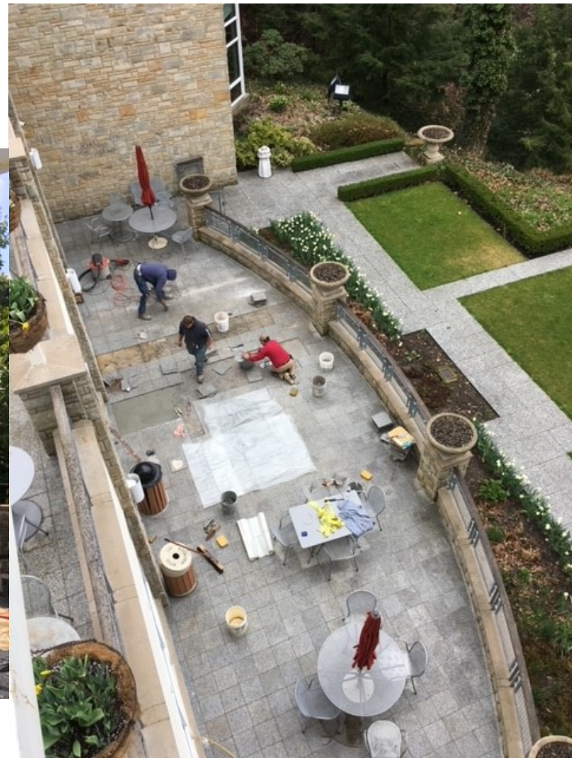
White Garden Terrace tile repair - 2017
