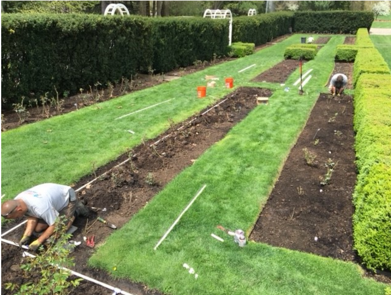
Rose Garden irrigation system renovation - 2017
