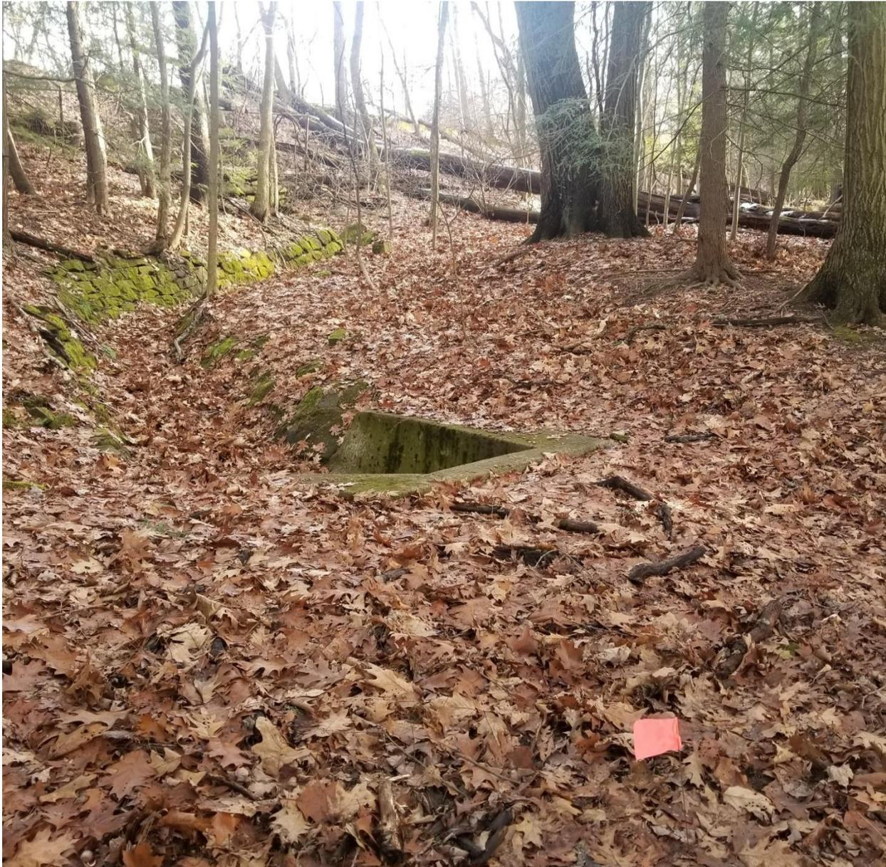
7. View of the east, showcasing an existing stormwater drainage as it approaches the previously mentioned culvert. The preferred alignment will utilize the existing culvert and will have no negative impacts to existing infrastructure.
