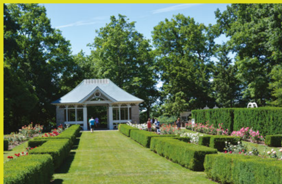
Kidston Pavilion in Fellows Riverside Gardens
